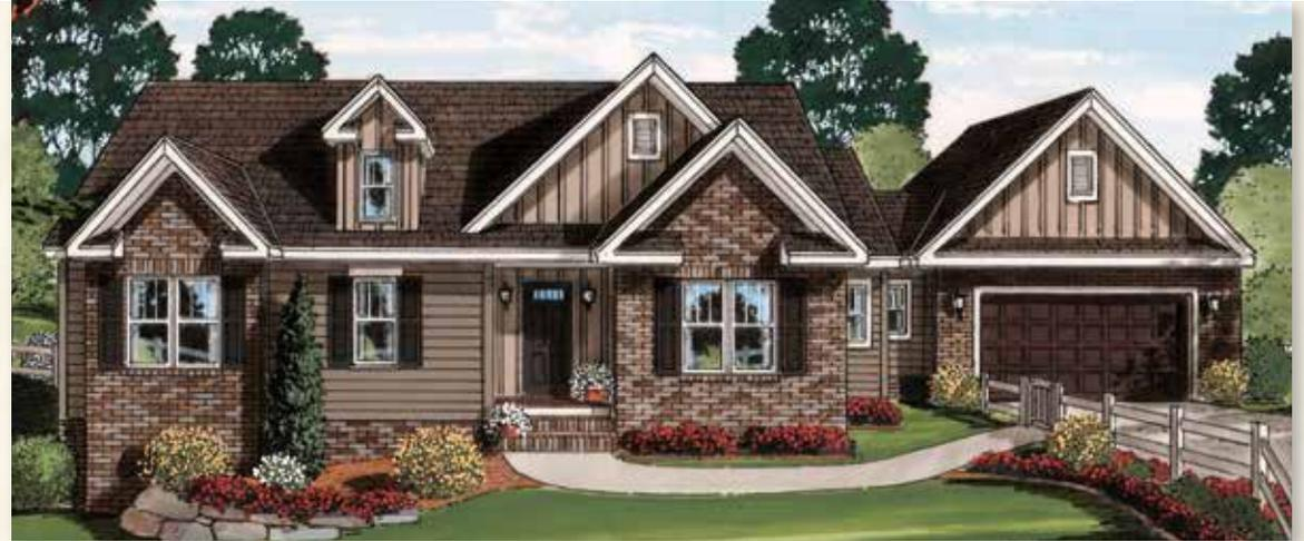
Shown with optional 9/12 pitch roof--standard roof for this plan is "tri-mod 7/12".
